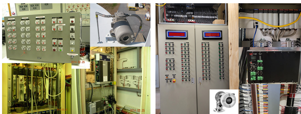
Figure 1. Previous control panel, PLC, servo gauge, and 8130 RTU (left), and new control cabinet, PLC, 8810 RTU, interior wiring/cables, and NMS81 Servo Gauge (right).
