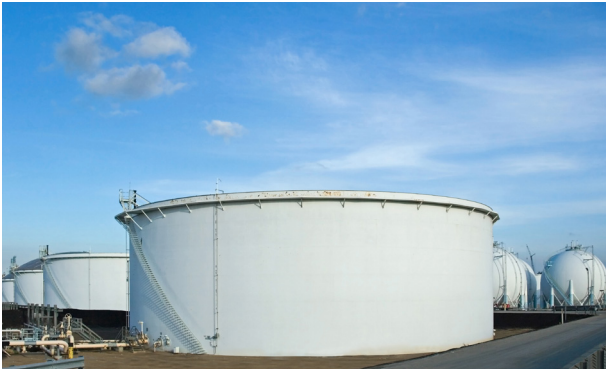
Figure 1. Bulk liquid tank farm.
