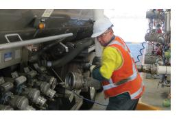
▶ Drivers are able to load using up to three Liquip® Load Arms simultaneously per bay. One bay provides two unloading arms for
