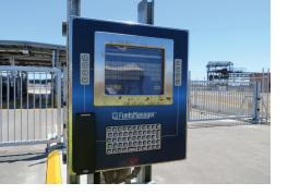
► The Varec Driver Entry Terminal interfaces to FuelsManager Oil & Gas Terminal Automation System to verify driver identity and control facility access.
