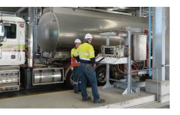
Each bay uses an FMC Technologies Smith Meter® AccuLoad® III to control injectors, flow meters, pumps and valves for blending, additive injection, and loading/unloading.
