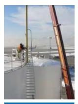
A radar operating without a stilling well needs to be installed away from the tank wall, where tank deformations have increased impact on its accuracy.
