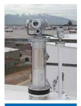
Installing AC/DC-powered roof reading instruments on a standard petroleum tank could easily add \$3,000 to \$5,000 in conduit costs.
