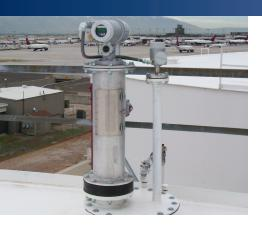
► The 6005 Servo Tank Gauge is ideally suited for jet fuel applications. It provides a high accuracy level measurement (+/- 0.7 mm), interface level measurements of up to three liquids, spot and profile density measurements and tank bottom measurement.
