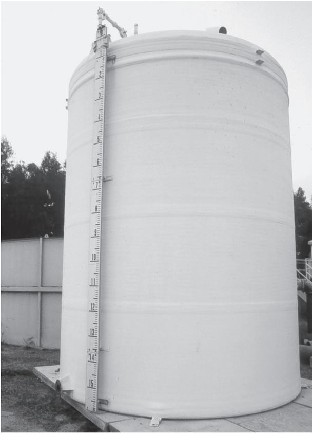
**Figure 1.** A gauge board on a tank.
