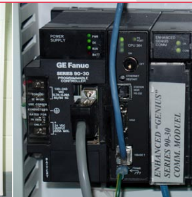
Existing programmable logic controllers (PLCs) were upgraded to the latest technology and interfaced to the base communications network
