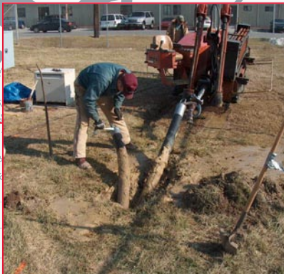
Single-mode fiber-optic cables were installed from the pumphouses to the base communications network
