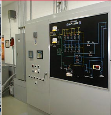
FuelsManager was upgraded and configured to communicate directly with the hydrant fueling system Control Panels
